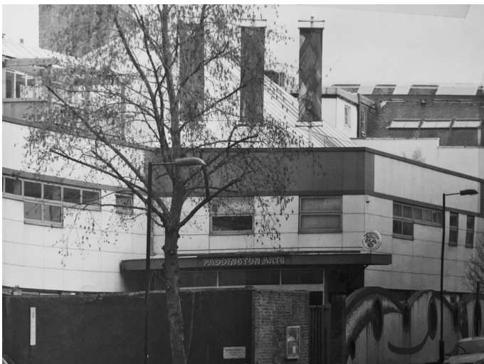
FIGURE 7.2 Paddington Arts building and performances.
