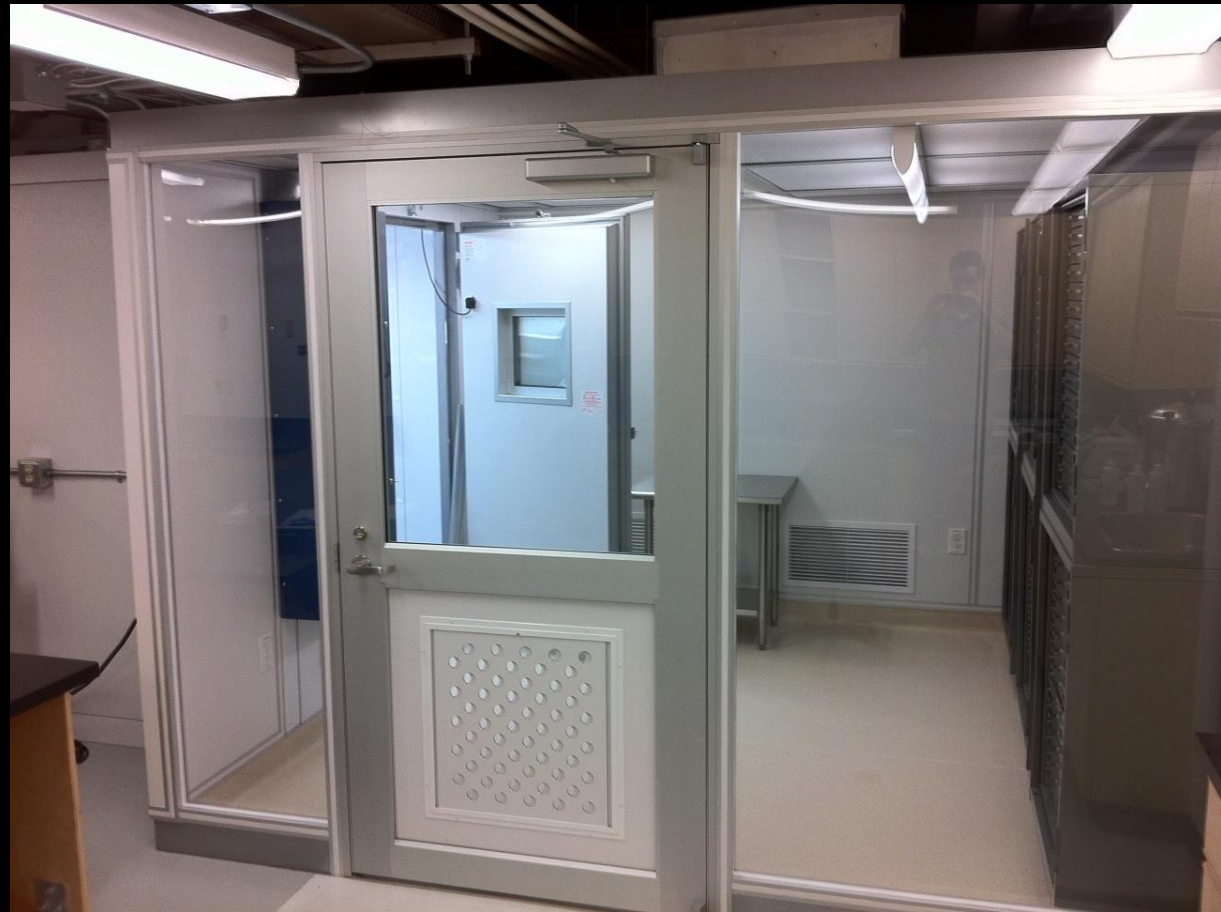
Class 1000 clean anteroom, with door to freezer (at left)
